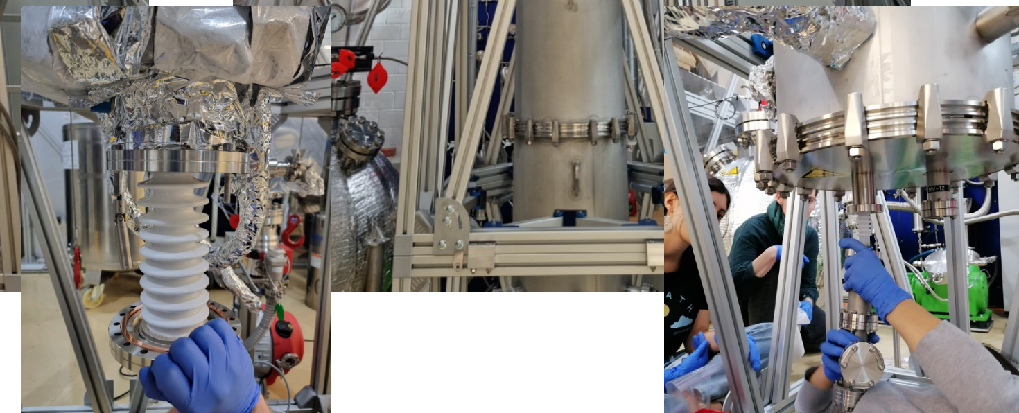
Close outer cryostat section by section, connect box, install HV feedthrough.
