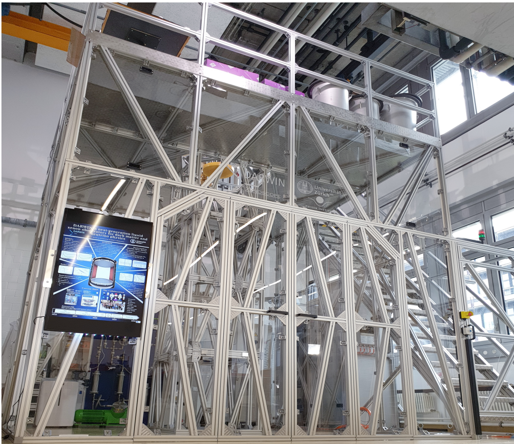
Figure 2.3.: Support structure of the demonstrator constructed at the assembly hall of UZH, Irchel campus. [51]
